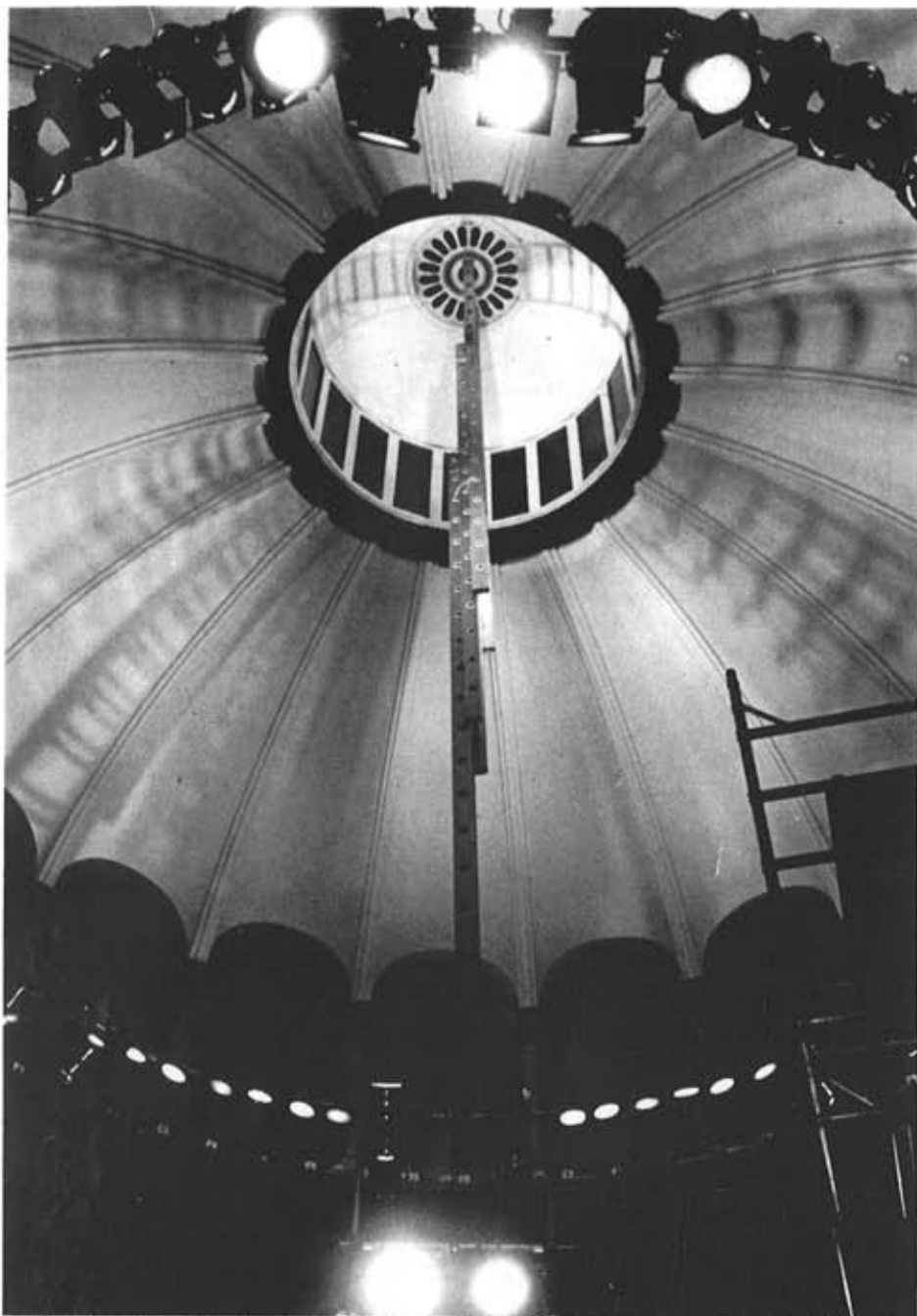
Looking up to the dome, showing part of the circular lighting rig and the suspended 3-part ladder.
