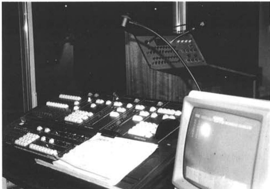
The MAC custom-built stage management console in the background, with the Strand Gemini lighting control nearest camera.
